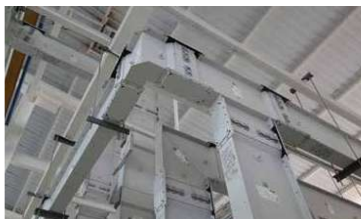
Example of Legrand busbar system
