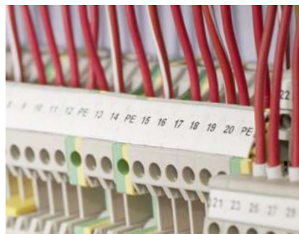
DEK/WS/MF: Flexible connector markers - print, clip, finished
